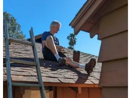
marks on it from its original use, but just enough rain had come down through it over time to damage the ceiling, so we took a closer look. After Gary sealed the coffee can to eliminate future leaks...the "historic" coffee can was kept in place.
